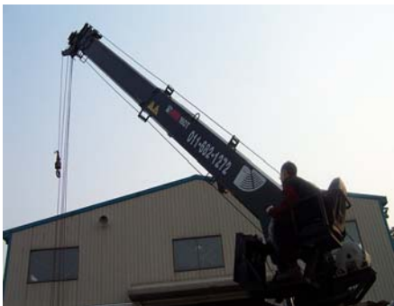
Figure 1.1 removal of wire rope
