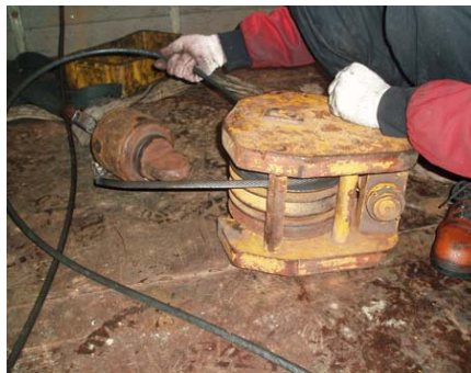
Figure 1.2 removal of hook
