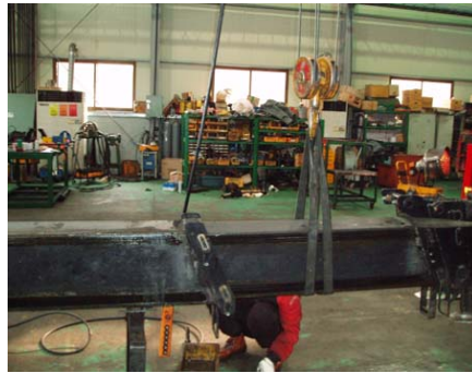
Figure 1.10 removal of 3 rd to 6 th boom
