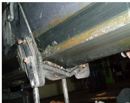
Figure 1.4 removal of sliding pads
