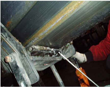
Figure 1.9 removal of sliding pads
