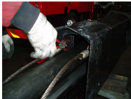
Figure 1.22 removal of retracting wire rope
