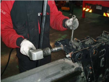
Figure 1.13 removal of adjusting nut of extending wire rope
