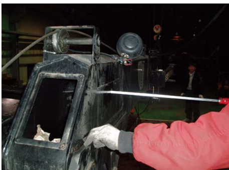
Figure 1.3 removal of ext. cylinder pin
