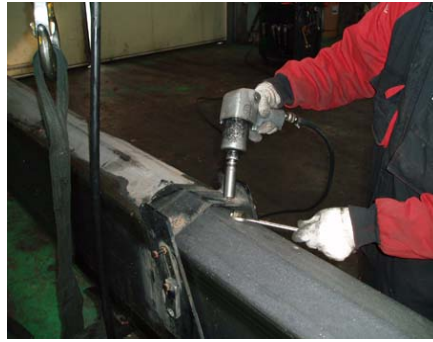
Figure 1.8 removal of adjusting bolts
